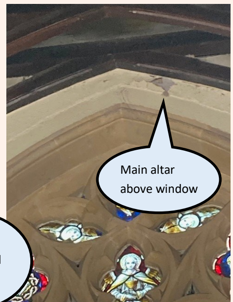
Choir loft cracking and peeling
