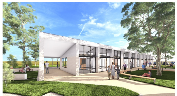
South West Corner View
